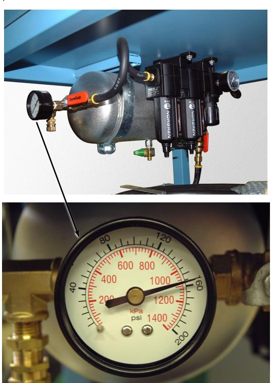
The regulator adjustment is located underneath the cart top shelf and next to the air tank assembly. To adjust, pull down on the knob to unlock for pressure adjustment.
