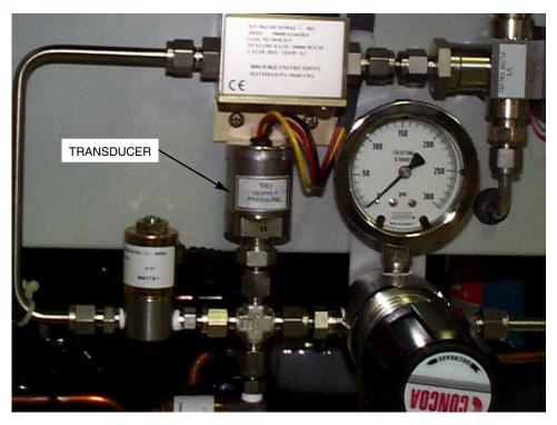
2) Insert the new transducer assembly as in the photo.
