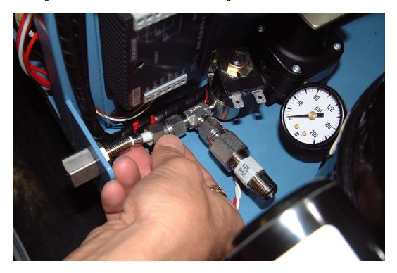
22. Reset the regulator pressure back to 150 psiG while the 2500 system is in the operating mode.
