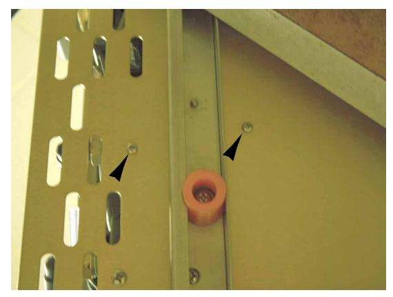
3. Remove flowmeter mounting screws, located on the underside of the unit.
