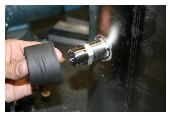
22. Remove the reservoir fill port assembly using an adjustable wrench.
