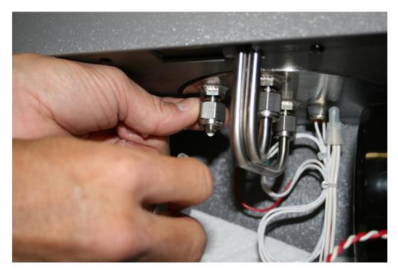
11. Make sure the tube is tight enough not to leak.
