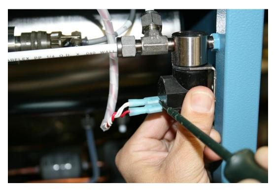
8. Using a large flathead screwdriver, remove the valve coil.
