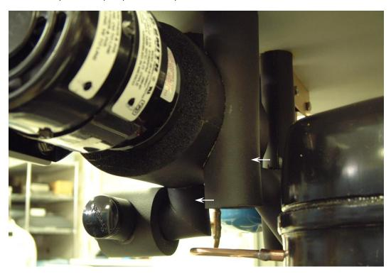
4. Drain the methanol from the system. Refer to the manual for methanol draining procedure.
