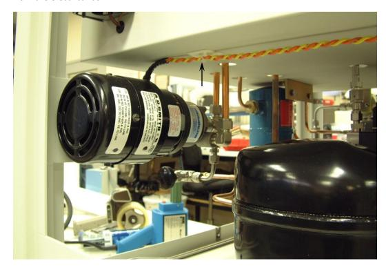
6. Remove the five screws from the fluid pump.
