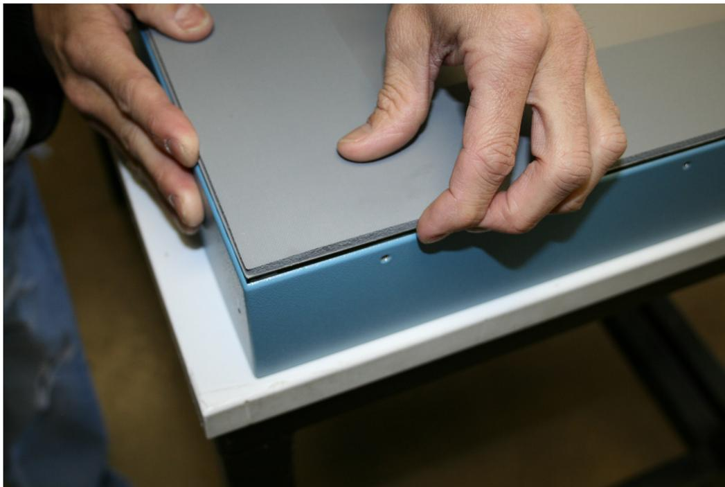
9. When final alignment is achieved smooth out the liquid. The gasket should dry thoroughly in 4 to 6 hours.
