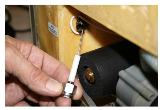
35. Inspect the probe for any build up on the Inconel metal part of the probe. Clean the probe using an emery cloth to clean it.
